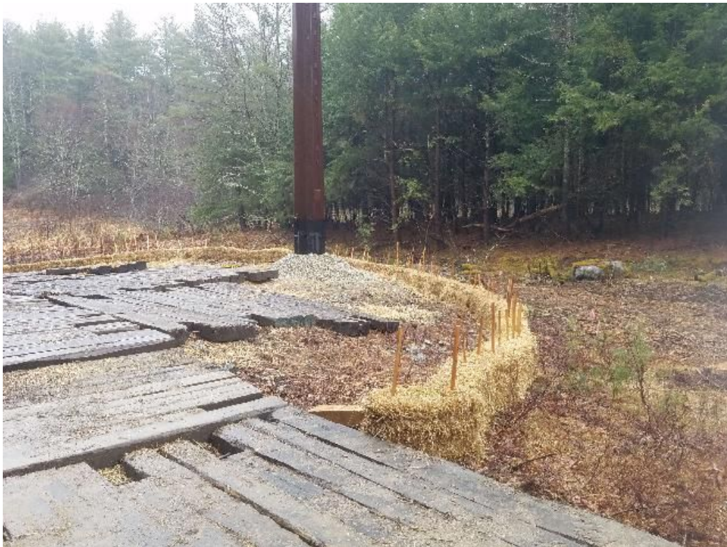
Fig 10: BMPs around Str. 68 work area and foundation. Viewing east. (04-03-20).
