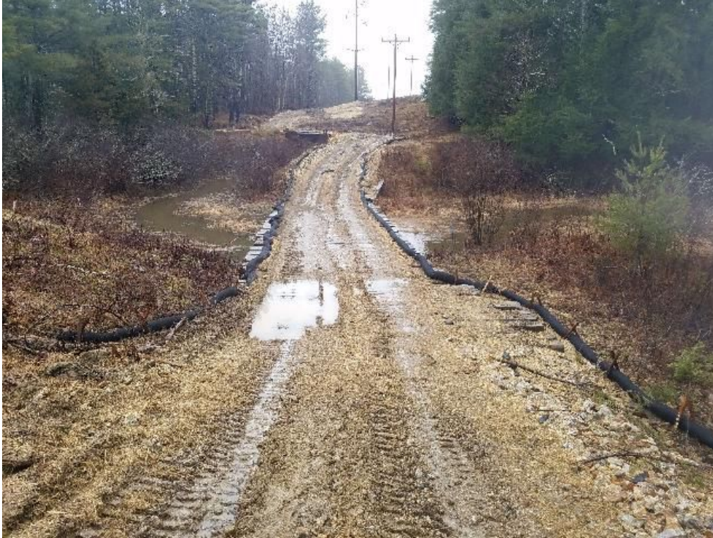
Fig 5: Access road between Strs. 51 and 52, over stream DS46. (04-03-20).
