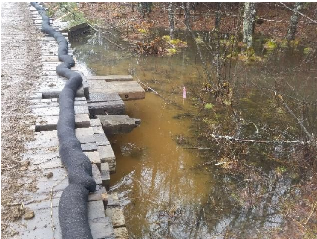
Fig 12: Access road between Str. 75 and 76. Note minor sediment through timber mats into wetland DW25. Viewing west. (04-03-20).
