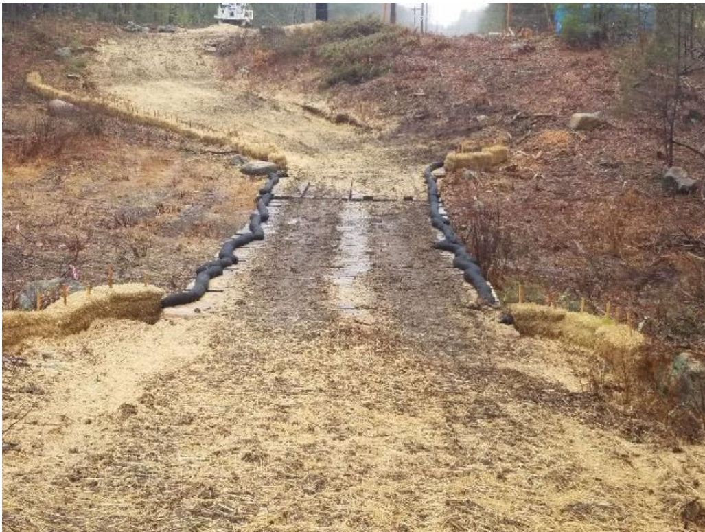
Fig 8: Access road through wetland DW9. Viewing west. (04-03-20).
