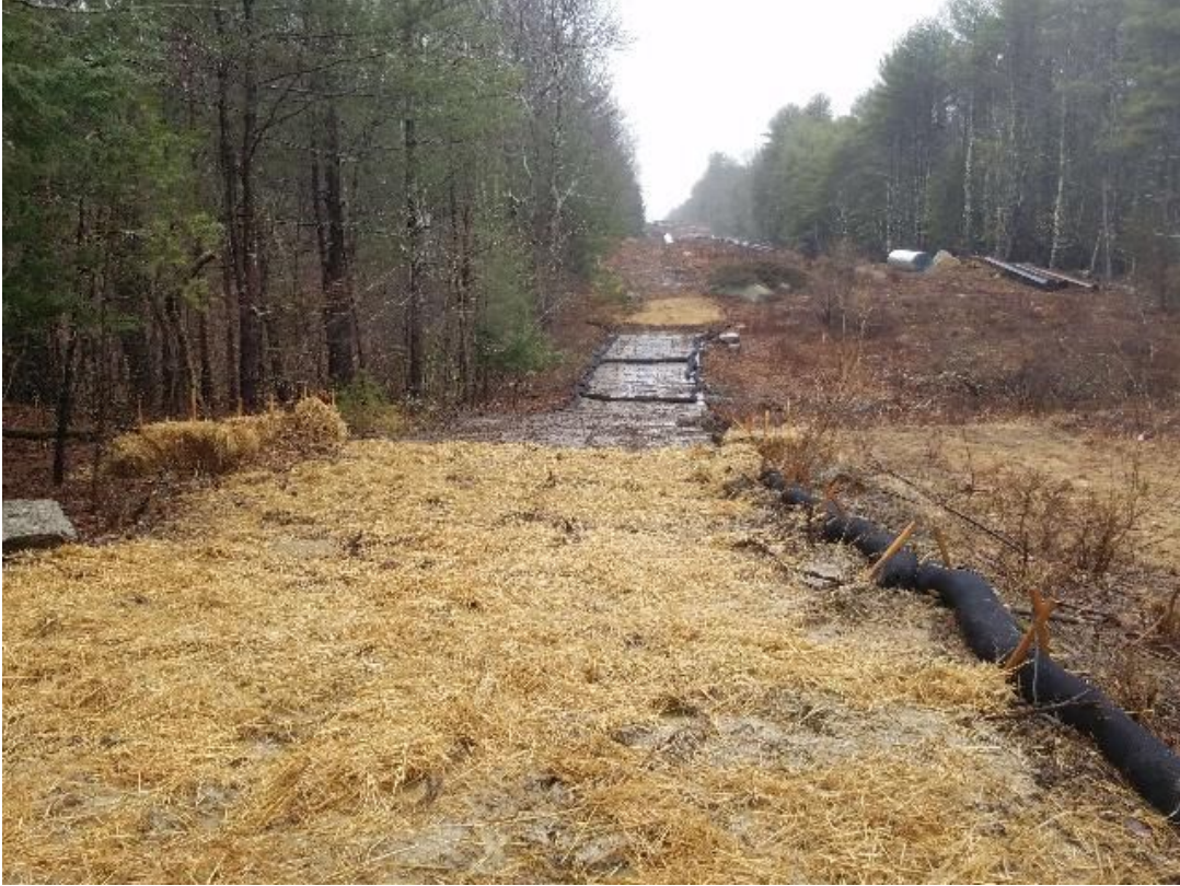
Fig 13: Access road from Str. 85 to 84. Viewing west. (04-03-20).
