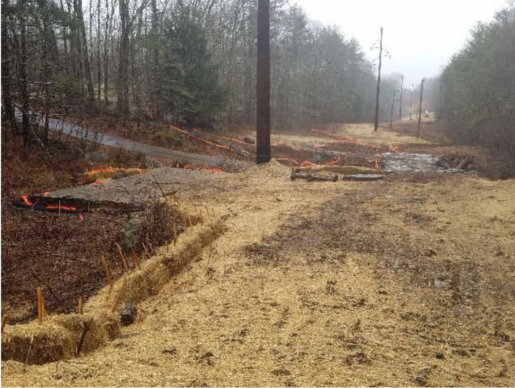
Fig 9: Str. 63 work area and foundation. Viewing west. (04-03-20).
