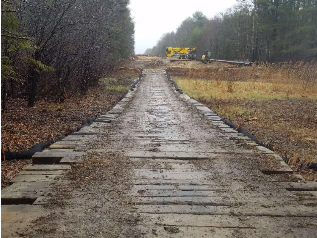
Fig 11: Access road through wetland DW21, between Str. 74-75. Viewing east. (04-03-20).
